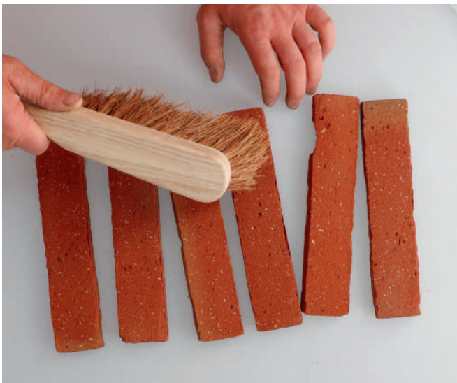
Dedusting the back side of the brick slip
