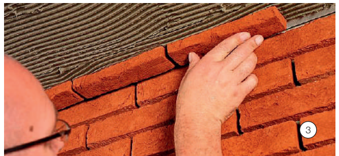
Installation of the brick slip
